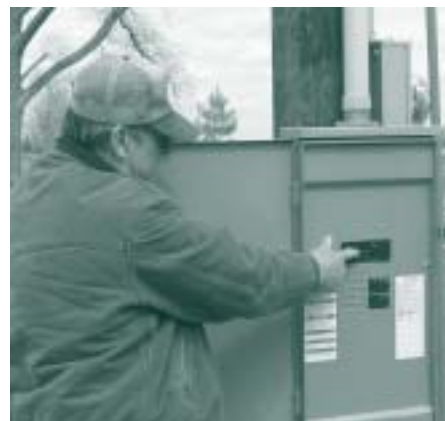
Hawkeye Marketing Representative Wayne Kirkeby pointing out the disconnect switch. On this type of device you reset it by pushing the switch to opposite position (off) and back again (on).
