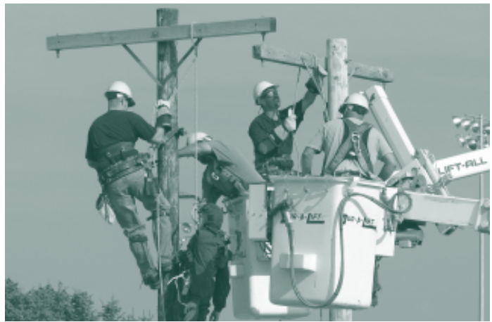
Hawkeye's Safety Coordinator, Mark Zweibohmer, inspects each lineman's tools (belts, gaffs, gloves, hard hats, safety glasses and more) for signs of damage or wear before they can start the testing procedure.
