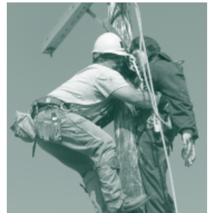
Lineman Jim Bakken wraps his hand line (rope) around the victim's body.
