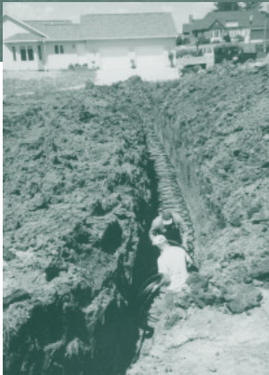
The Frana's home required a six ton unit and a lateral underground loop system.
