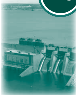
Flambeau Hydroelectric Station
