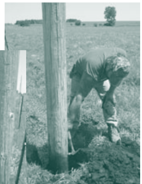
Ameripole Inspection Company checks, evaluates and treats utility poles on a seven-year rotation.
