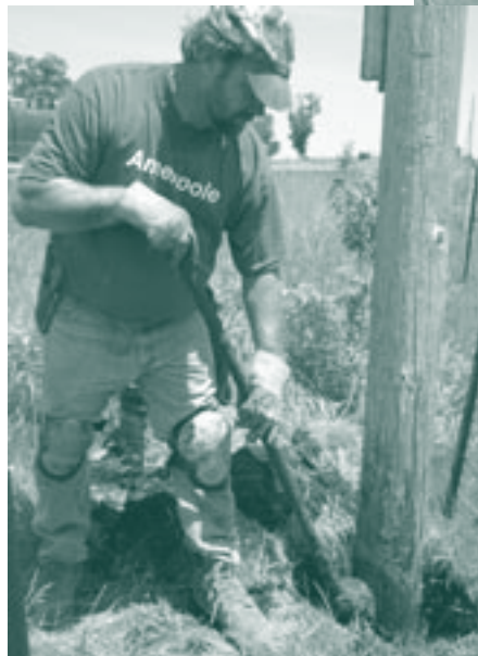
Ameripole Inspection Company checks, evaluates and treats utility poles on a seven-year rotation.
